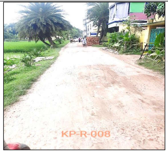
Road-08, Keshabpur Paurashava
