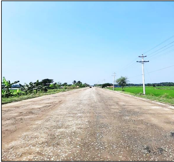
Road-01, Keshabpur Paurashava
