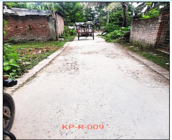
Road-09 , Keshabpur Paurashava
