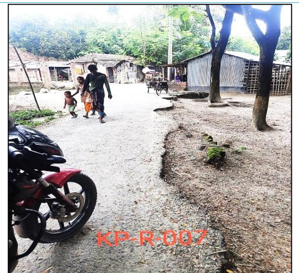
Road-07, Keshabpur Paurashava
