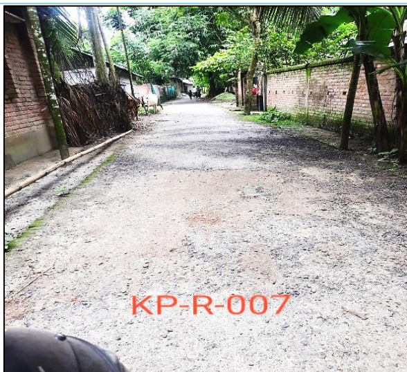
Road-07 , Keshabpur Paurashava
