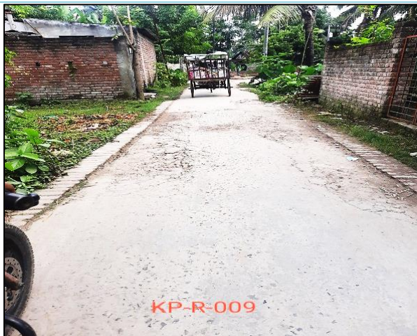
Road-09 , Keshabpur Paurashava
