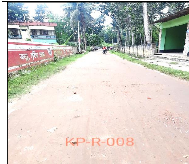
Road-08, Keshabpur Paurashava
