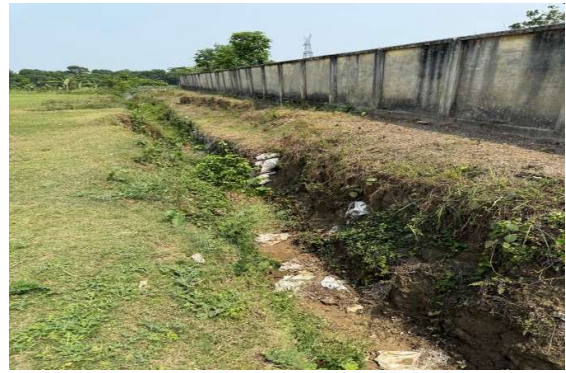
BHER -D-05: Construction of RCC drain starting from Farakpur Near Grage Field to Borokol Khal (Ch.185.00-25.00m) in ward no. 02 under Bheramara Pourashava, Kushtia.
