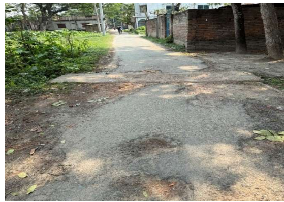
BHER -R-23 Construction Construction of Nawda Para Sub-Zone Road starting from near Nawda Para Sub-Zone Mosque to near Principal Rejaul House by RCC (Ch.0.00 to 144.00m), including 01 no. Cross Drain at Ch.83.00m
