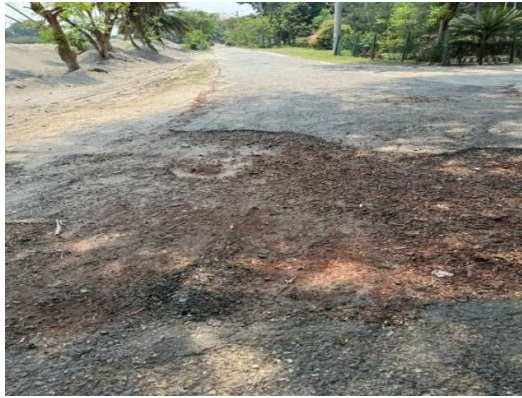
BHER-R-04 Rehabilitation of Road starting from Frakpur Hospital Road to water Board Last boundary by DBC (Ch.0.00 to 815.00m) and Link: starting from Bot-tola to MP road by DBC (Ch.0.00 to 168.00m) & Installation of 34 nos. Street Light in Ward no. 02
