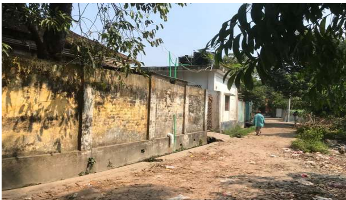
BP-R-07: Improvement of road by Dense Bituminous Carpeting (DBC) at T.A road, starting from Kazipara Dhopabari mour to Moulovi Hati Masjid to Gukorno road. at Ward no - 8, Brahmanbaria Paurashava,
