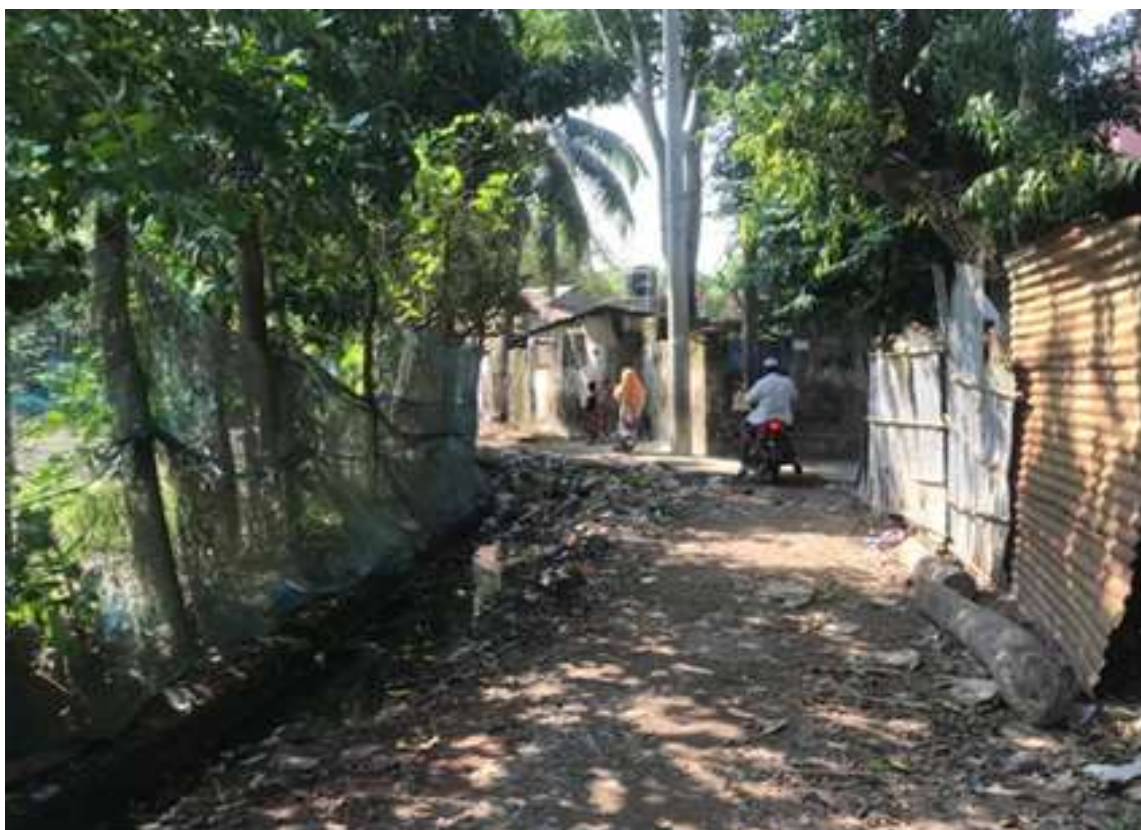
BP-D-22: Construction of RCC Drain at Kazipara, (a) starting from Dhobabari mour to Town Khal at Ward 8, Brahmanbaria Paurashava, Brahmanbaria
