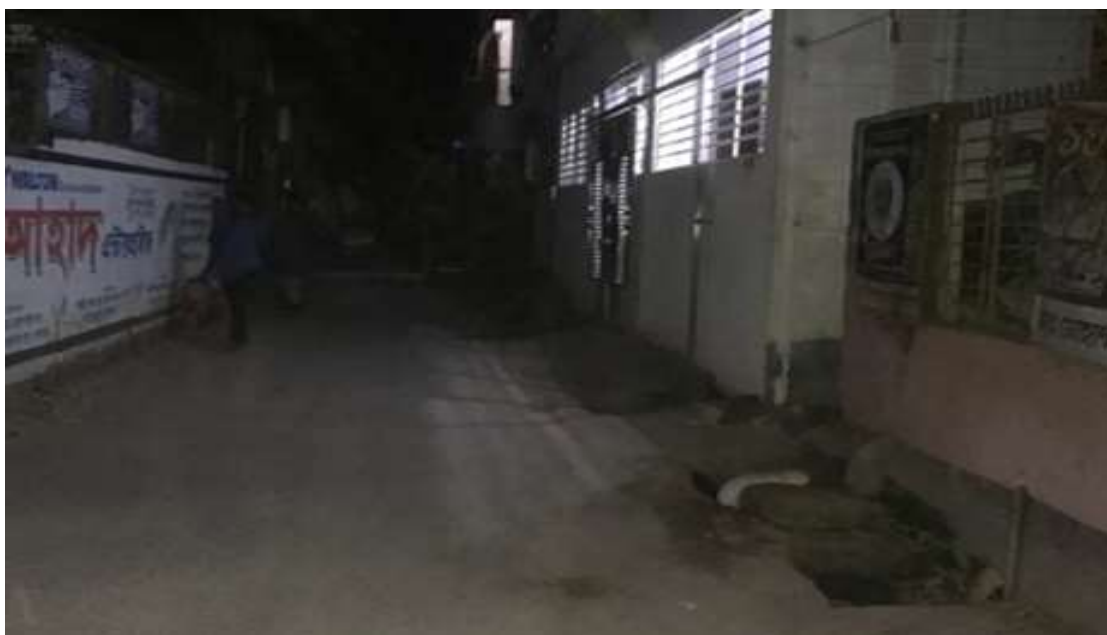
BP-D-005: Construction of RCC drain (a) at Purbo Paikpara Dhopbari road starting from Cumilla-Sylhet Road to Proposed Drain 5(b) via Daspara Primary School (b) at Gogon Saha Bari road starting from Cumilla-Sylhet Road to Titas River at Ward no - 04, Brahmanbaria Paurashava, Brahmanbaria
