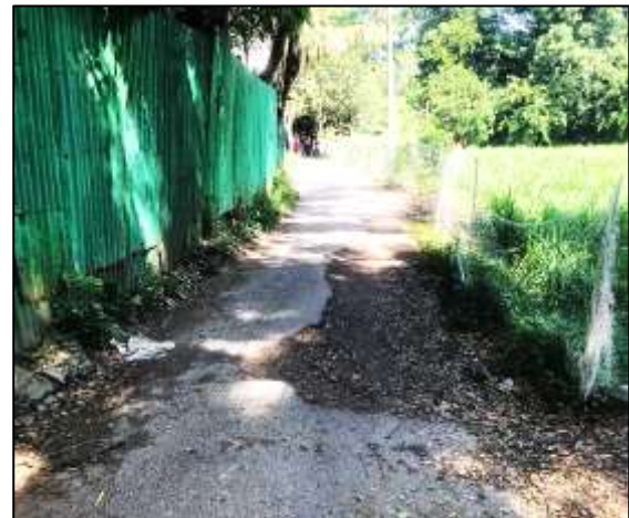
CP-R-240: Improvement of Road by Dense Bituminous Carpeting from Barkal Shark to Khanhat (Cox's Bazar Road) at Ward no. – 09, Chandanish Pourashava.
