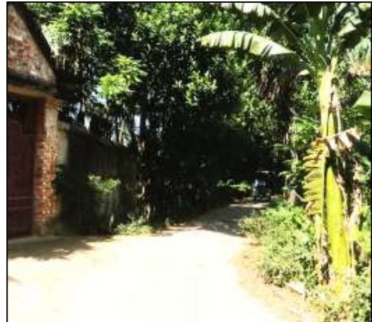
CP-R-137: Improvement of Road by Dense Bituminous Carpeting from Noya Hat Road via Jihos Fakir para to Abdul Bari Hat at Ward no. – 06, Chandanish Pourashava
