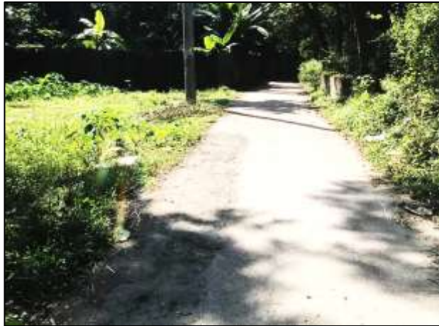
CP-R-45: Improvement of Road by Dense Bituminous Carpeting from Barkal Road (Sogir Mohammad) via East Chandanaish to Chowdhury Para at Ward no. - 02 & 07, Chandanish Pourashava.
