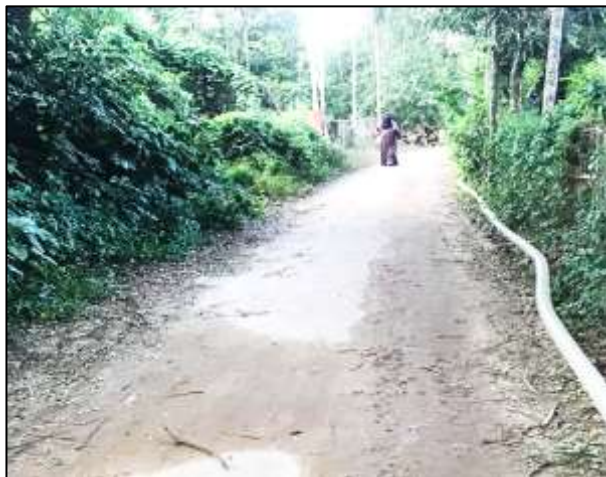
CP-R-169: Improvement of Road by Dense Bituminous Carpeting from Mawlana Ishak Road via Barkal Road (Mirjir Dokan) to Rahamaniya Bridge at Ward no. - 02, 05, 06, 07, Chandanish Pourashava.
