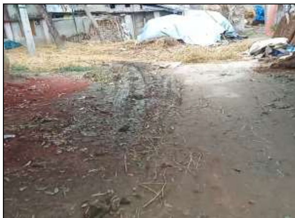
NAOH-R-03: Rehabilitation of DC Road by Bituminous Dense Carpeting from Naohata Bagata Poshu Hospital to Paikpara to Naopara Madrasah including Protection Work at Naohata Paurashava, Rajshahi.
