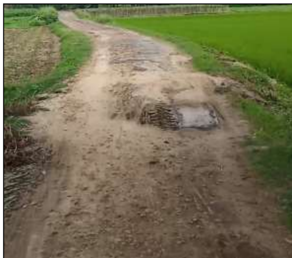
NAOH-R-59: Rehabilitation of Road by Bituminous Dense Carpeting from Puthiapara Ansar Camp RHD Road to Modunhati Government Primary School including Protection Work at Naohata Paurashava, Rajshahi.
