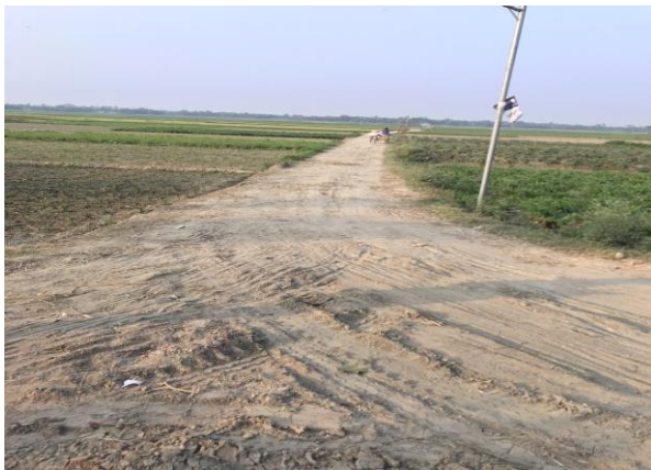
SP-R-07: Improvement of Earthen Road by BC at Boilmary Koborstan to Chomorpur Canal including Cross Drain under Santhia Paurashava, Pabna. (Length=1450m)
