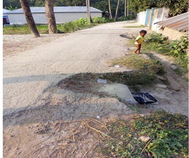
SP-R-05: Improvement of BC Road from Shalghor Hanu's Shop to Azahar-Afser Road including Protection work under Santhia Paurashava, Pabna. (Length=1572m)
