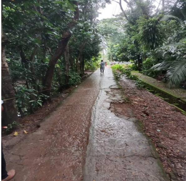
Photo SP.RD8.001: Improvement of Road starting from Hanif Mansion and ending near Johir Uddin Shimul road (Ch.0+00km to 0+490km) by RCC, including Protection work 20m at with 17 nos Street Light at ward no-08 under Sonagazi Pourashava, District Feni; Total Length = 490.00m.
