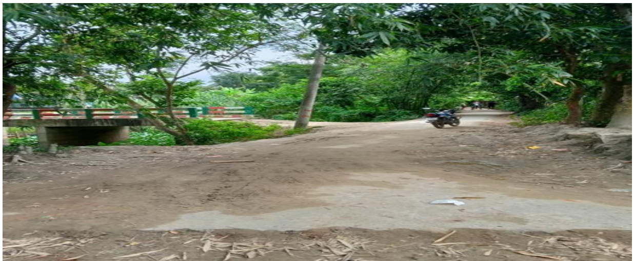
Photo SP.RD1/4/5.001: Improvement of Road starting from Mahbub Chairman Bari Road and ending near Main Uddin Bari (Ch.0+00km to 0+515km) by RCC & (Ch.0+515km to 0+765km) by UNI BLOCK, including Protection work 109m with 26 nos. Street Light at ward no-1/4/5 under Sonagazi Pourashava, Dis-Feni. Total Length = 765.00m.
