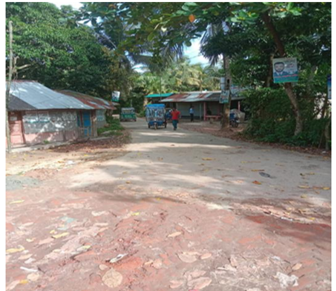
Photo SP.RD2.001: Improvement of Road starting from Doctor Mansion and ending near Boro Bari (Ch.0+00km to 0+305km , Ch.0+771km to 0+980km ) by RCC Road & (Ch.0+305km to 0+771km) by DBC, including Protection work 112m with 33 nos. Street Light at ward no-02 & 03 under Sonagazi Pourashava, Dis. Feni; Total Length = 980.00m.
